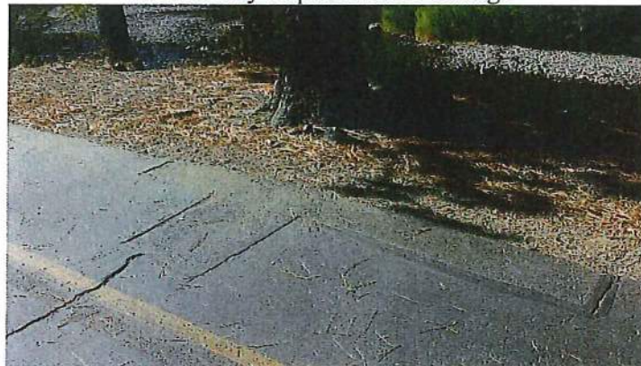
Previously Repaired Root damage
