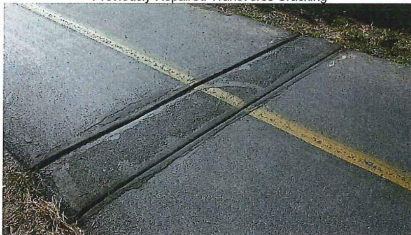
Previously Repaired Transverse Cracking
