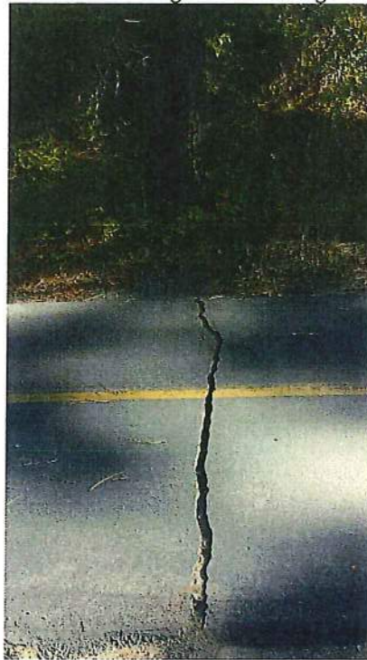
Previously Repaired Root damage
