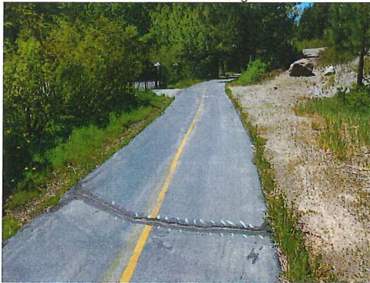
Previously Repaired Transverse Cracking
